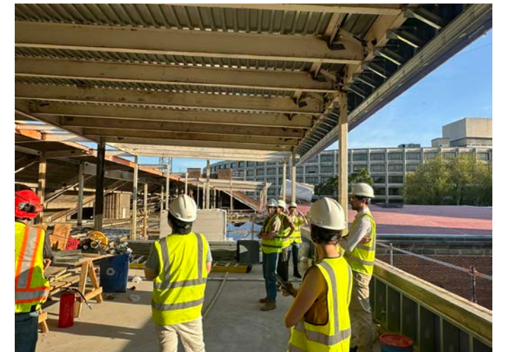
September 2024 New dormer floor poured & Roof decking installed
