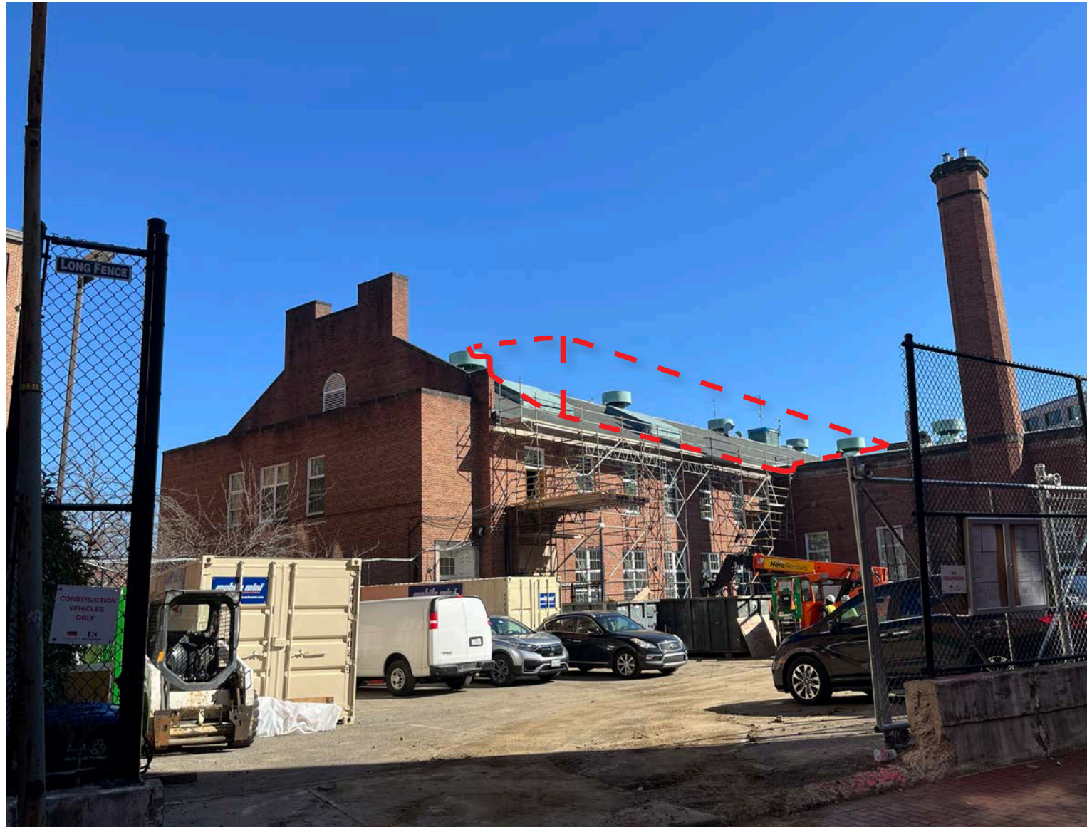
Rear, Before Roof Demo
