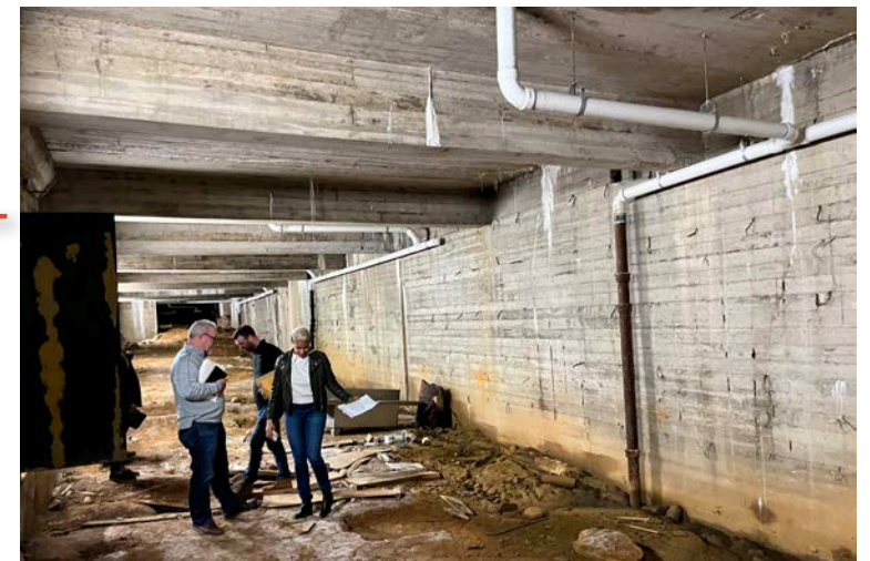
Former 'Crawl Space'
