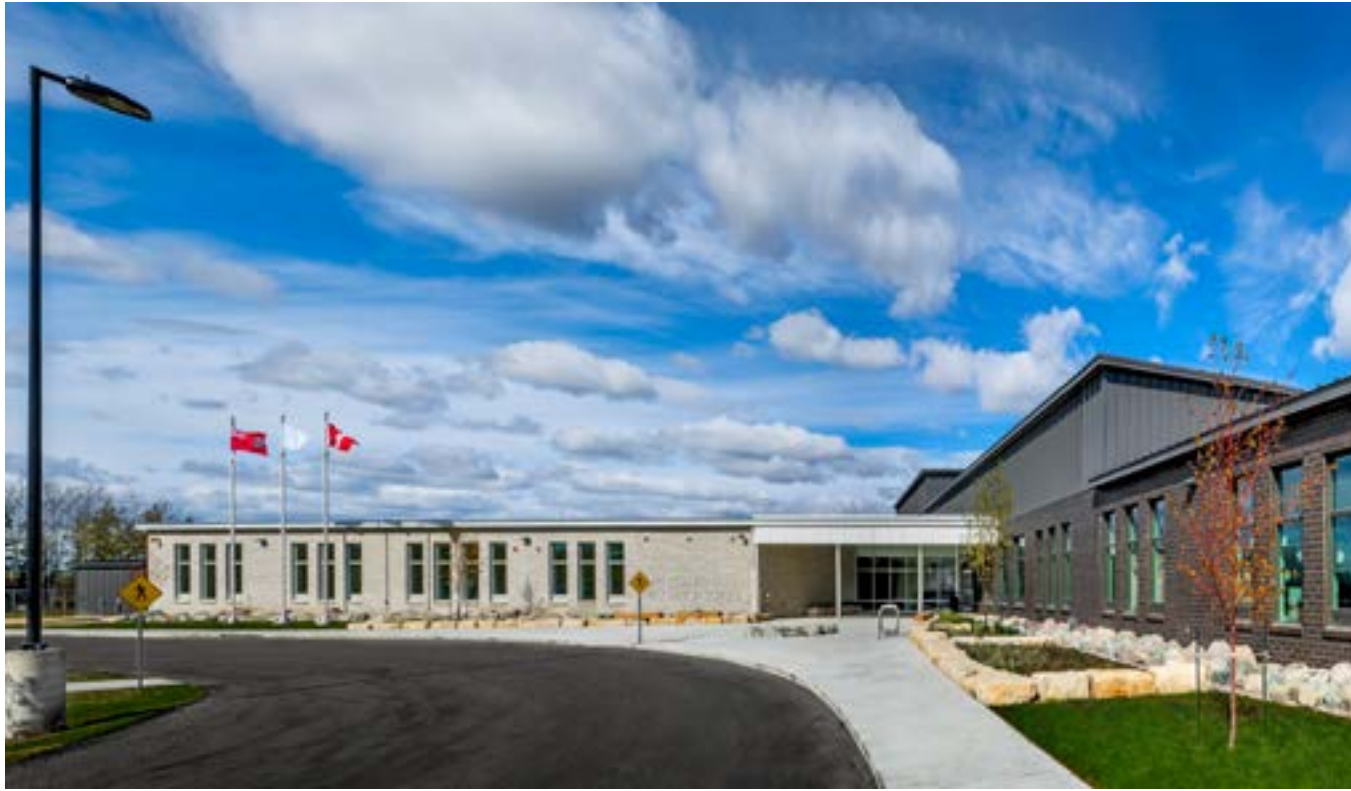
Main entrance of school
